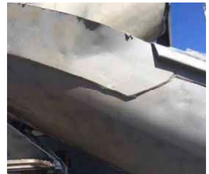
The same chute after the concrete was blasted off with the EcoQuip EQ400t.
