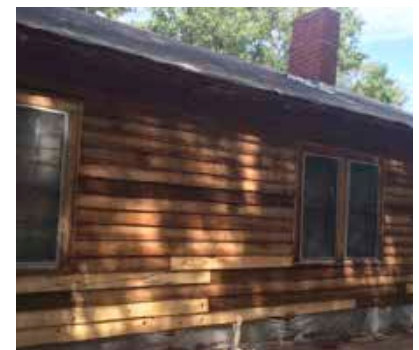
After the paint was removed from the home, the plastic used to catch the residue was easily rolled up and disposed of properly.
