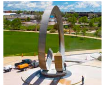
Very little containment is needed when blasting with EcoQuip 2 Vapor Abrasive blast equipment.
