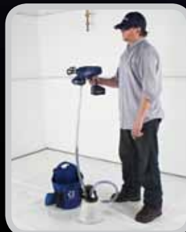
3. Turn on air compressor. Prime sprayer.
