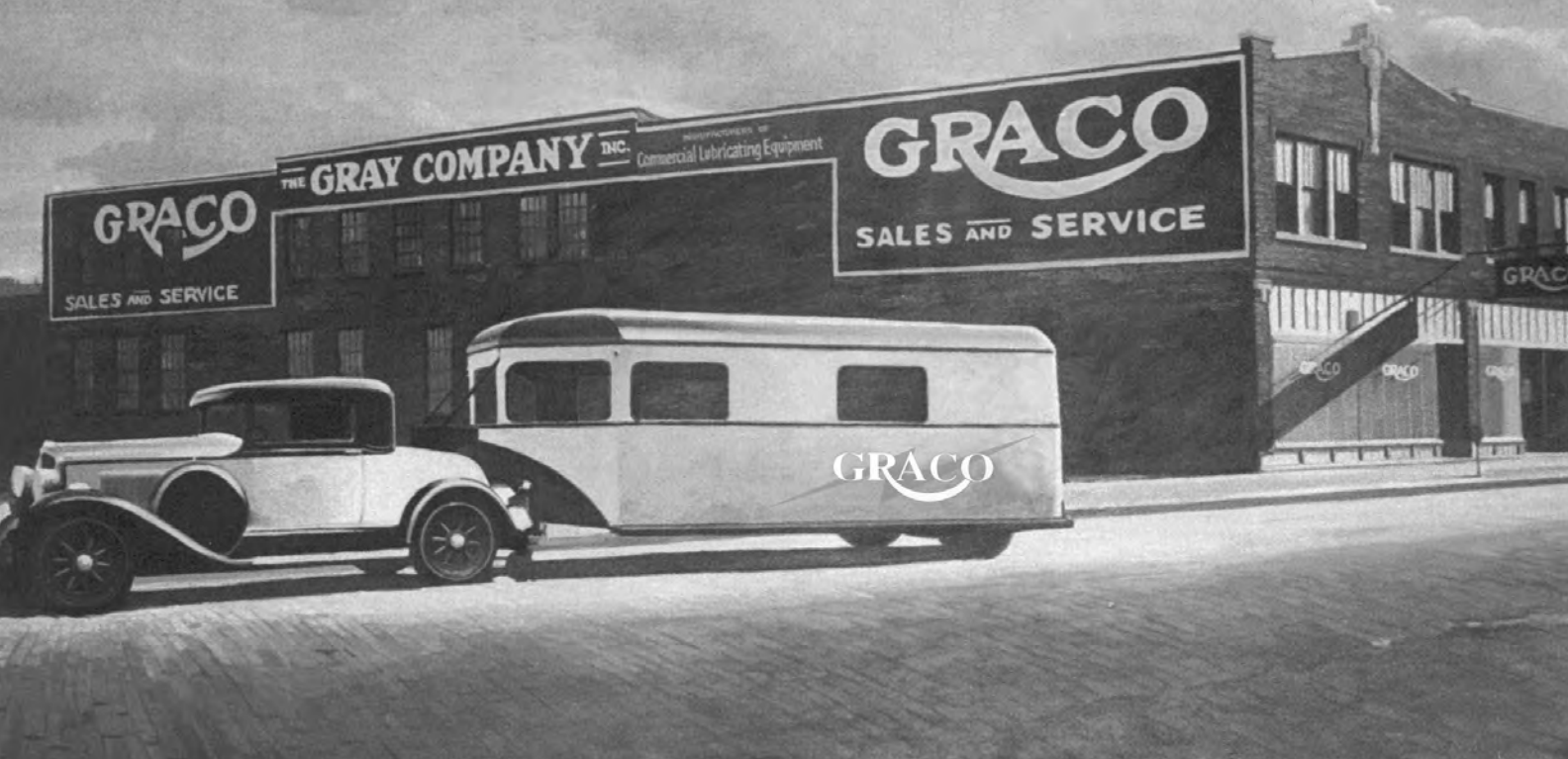
Traveling display outside Graco's first 1926 facility.
