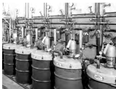
Industrial paint room installation featuring Gray Co.'s Power-Flo® paint supply pumps.
