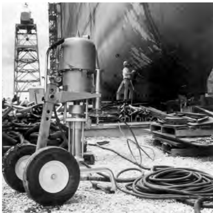
20:1 King® unit applying primer onto ship hull.
