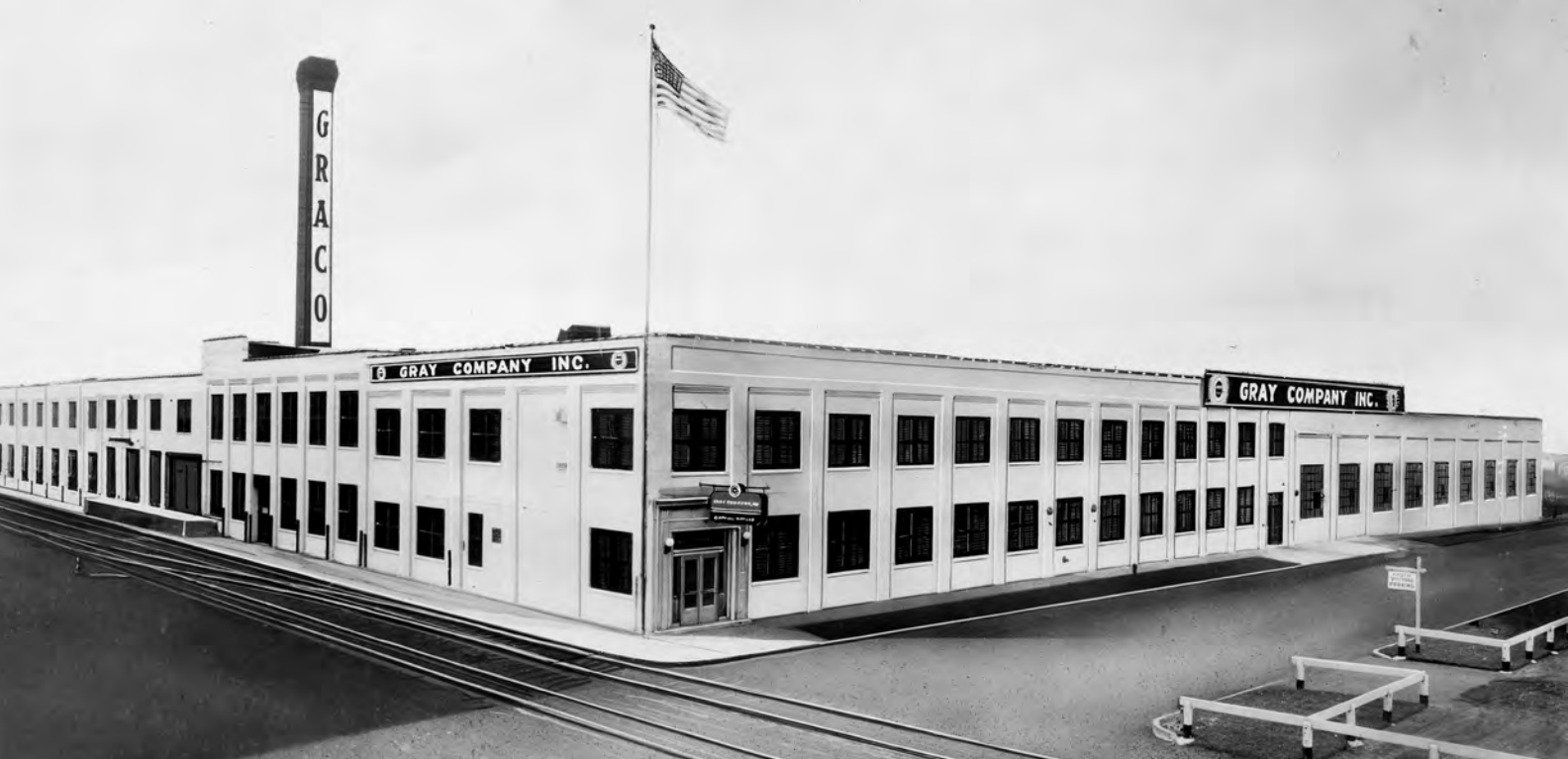
Graco's 60 - 11th Avenue N.E. manufacturing facility, circa 1945.
