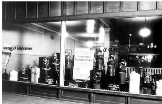
Equipment display window at 120 South 10th Street, Minneapolis, MN.
