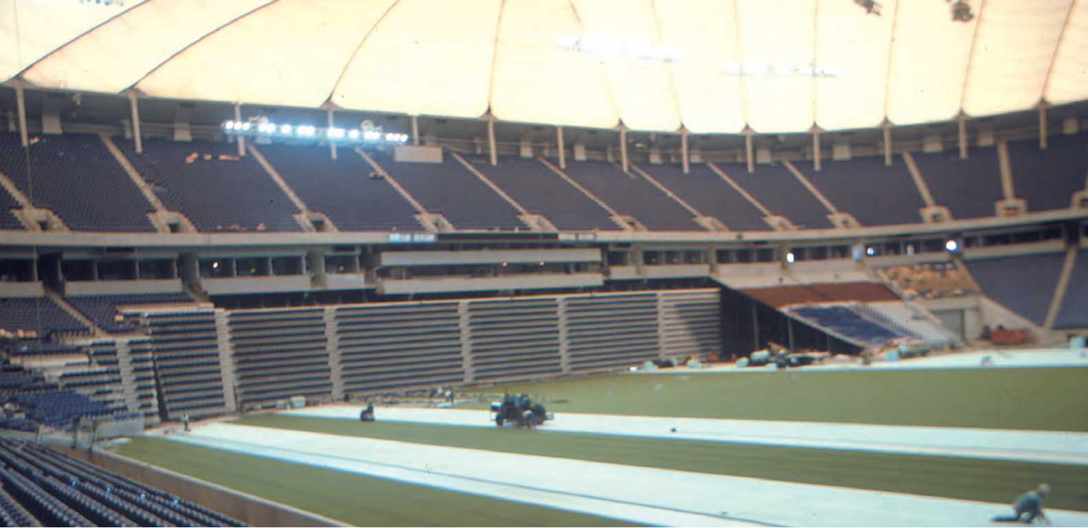
Graco's automatic airless spray guns applied adhesives between layers of foam rubber padding and turf at the Metrodome sports facility in Minneapolis, MN.
