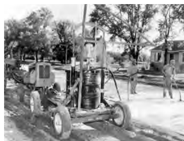
Mogul® high pressure extrusion pump on ram applying heavy sealing materials to roadway.
