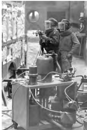
Hydra-Cat® - Graco's first plural component spraying unit is shown spraying foam insulation.
