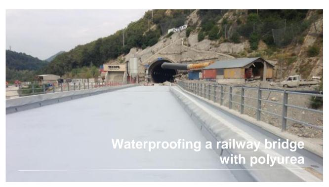
In this story, we describe the transformation of a concrete bridge used for the railway that needed to be coated with more than 6.000 m² polyurea. The bridge showed some damages and general lesions due to exposure to the elements for over 50 years with, as a consequence, cracks and water seepage in certain areas.
