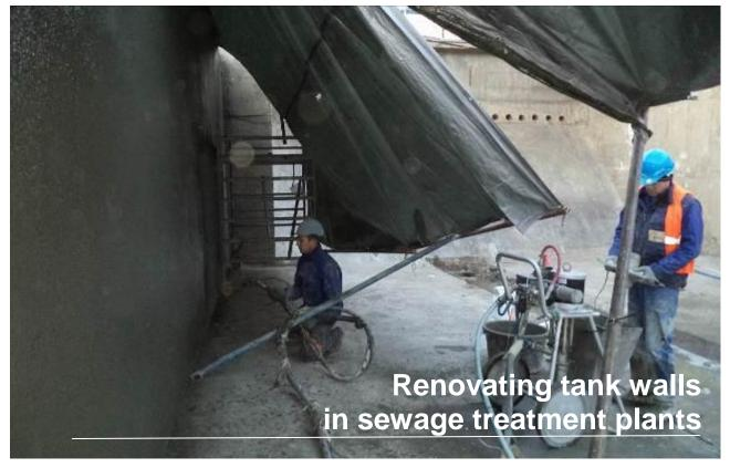
A contractor was assigned the renovation of secondary containment tanks at the sewage treatment plant in Tomaszów Mazowiecki, Poland. The old concrete and its surface protection had to be renovated due to waste water deterioration. The surface to be renovated was 2000 m<sup>2</sup> and the job was carried out in three phases.
