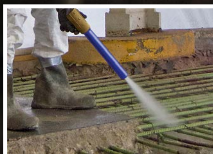
Concrete Repair and Restoration
