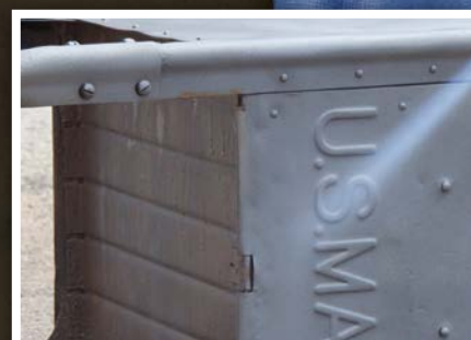
Steel Surface Preparation
