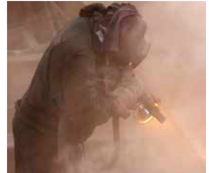
Standard sand blasting produces an excessive amount of dust and harmful particulates.
