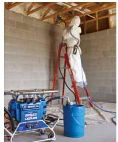
*The Reactor E-8p is the best choice for portability and high-quality spray foam since it's lightweight and compact at 95 pounds, and can be plugged into one 115V outlet.*
