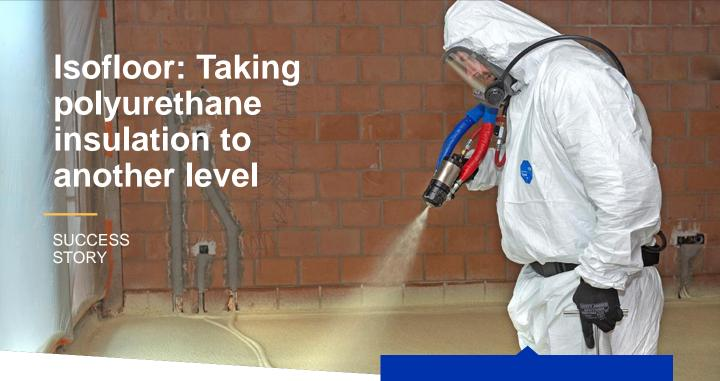
Belgian company Isofloor has been using Graco Reactors since 2007 to spray polyurethane insulation foam on all types of floors.
