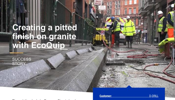
The existing kerb in Denman Street, London, UK, was causing damage to a range of high-class vehicles including Bentleys, Rolls-Royces and Jaguars that frequently pulled-up there to drop-off hotel customers. The kerb needed to be modified to prevent additional damage and a cycle path added. However, the modification of granite kerb stones is a time-intensive expensive process which usually involves road closure and a large amount of waste generated to create the desired effect.
